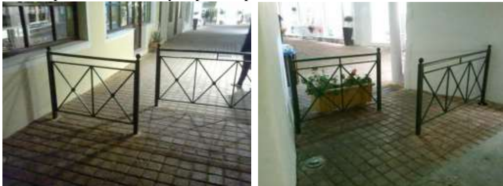
Figure 14,15: Tackling motorcycle moves while letting pedestrian, cyclists and wheelchairs to access the relieved zones.
