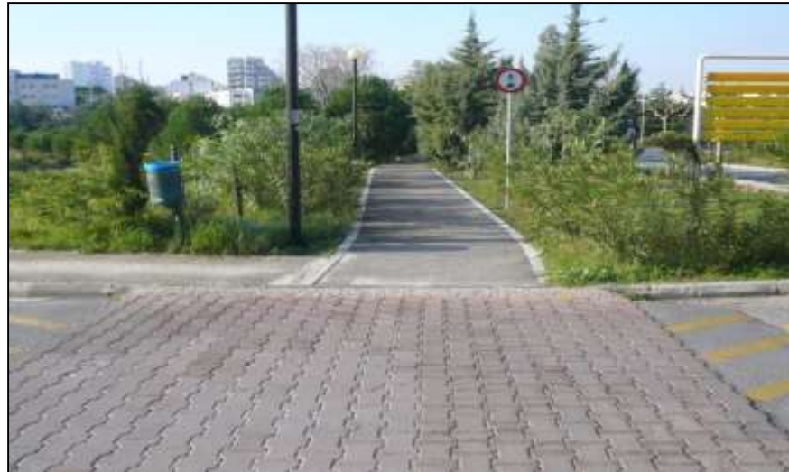
Figure 11: Image of the completed cycle lane inside the NTUA campus Source: Authors' archive
